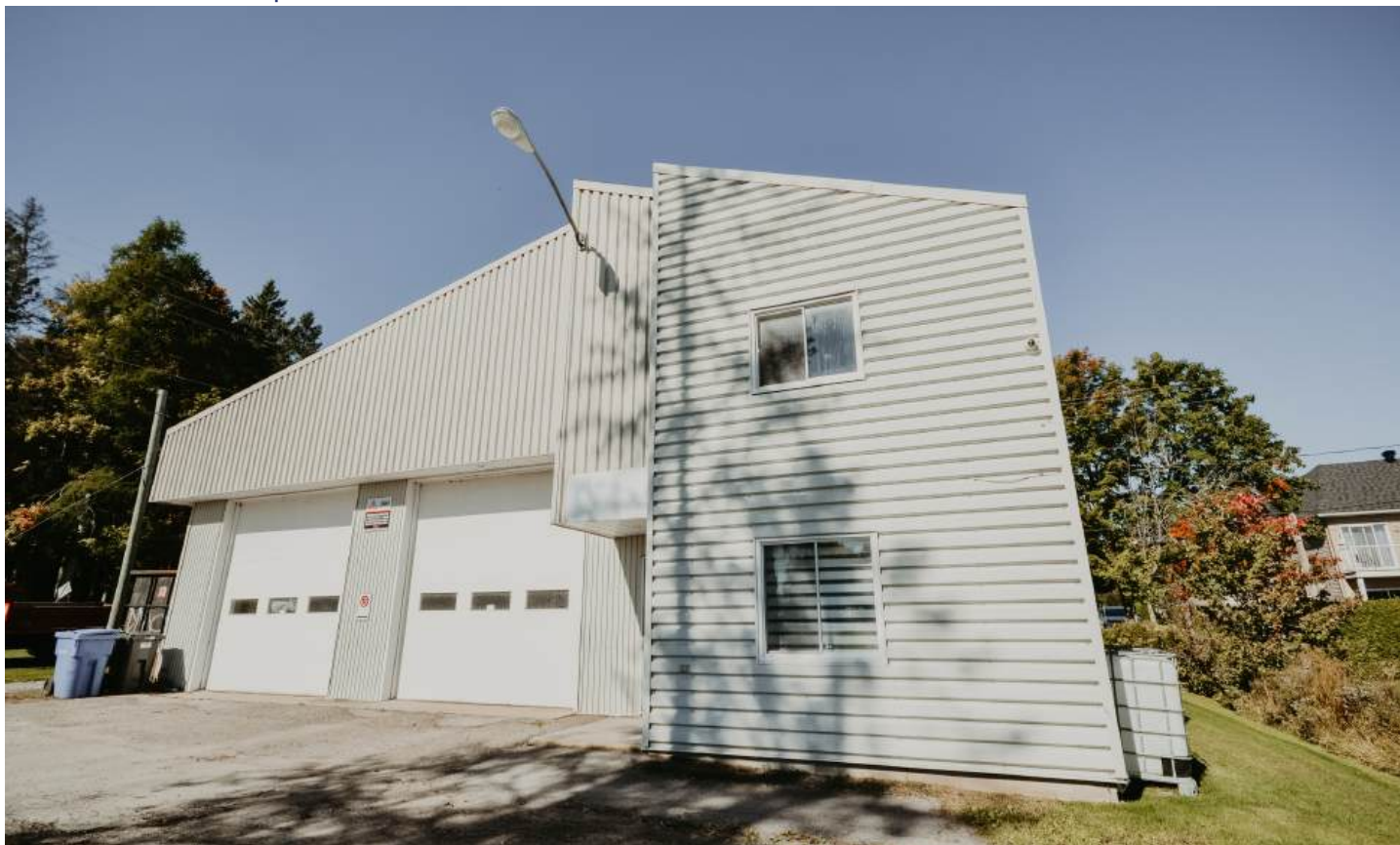
GARAGE MUNICIPAL (730, RUE OMER-BOUCHER)
